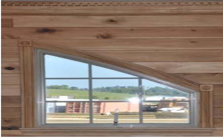
1X6 POPLAR FLOORING USED ON A WALL WITH POPLAR CASING & ROSETTES
