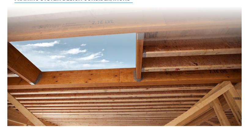
onCENTER® BLI joists provide the floor system designer several alternatives regarding joist series and depths. Exploring these options along with joist spacing should enable the designer to determine the optimal floor with consideration to the satisfaction of the end-user and the costs associated with the selection.
